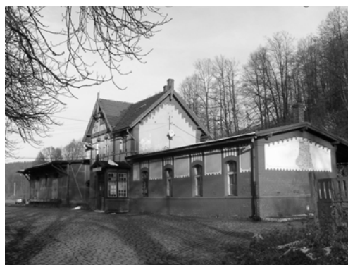
Fot. 3. Dworzec w Jugowicach. Photo. 3. The Railway station in Jugowice.
